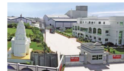
AGL Dapur Plant (GVT)
