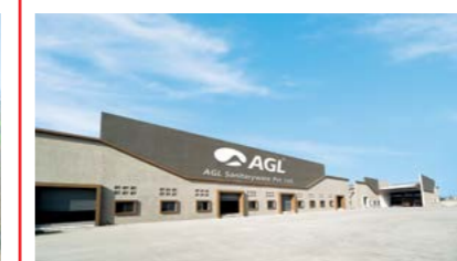
AGL Sanitaryware Plant
